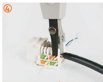
④ Impact & cut wires
