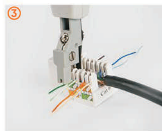
③ Pushing the wires into keystone jack
